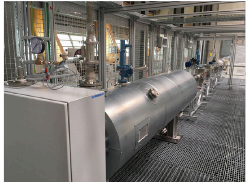
BACS build-up within safety fence
